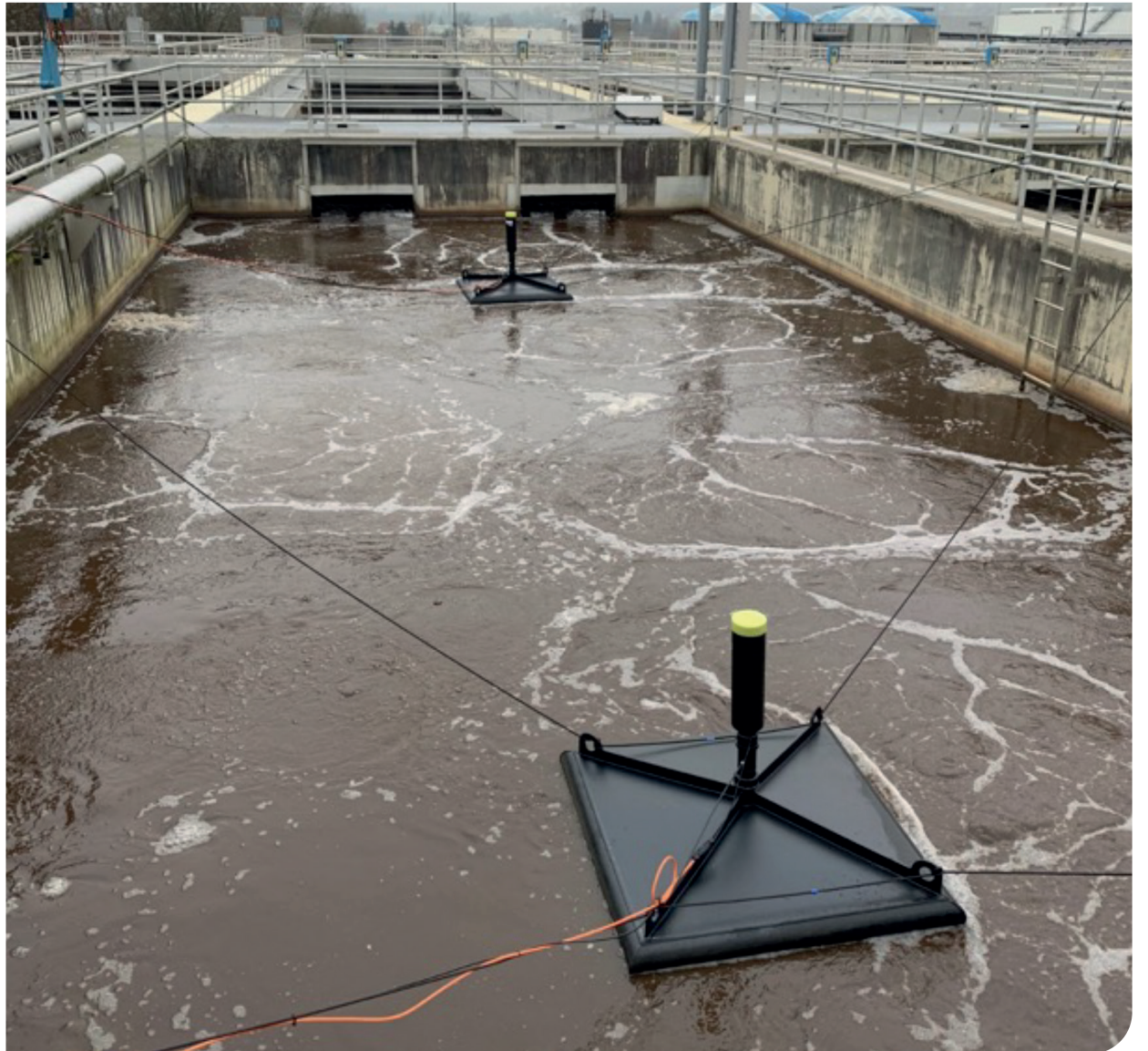
Municipal wastewater treatment plant
